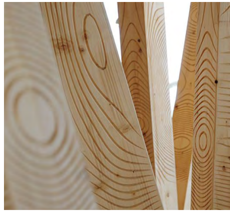
timber detail of the Monte Rosa Hut by Gramazio Kohler
