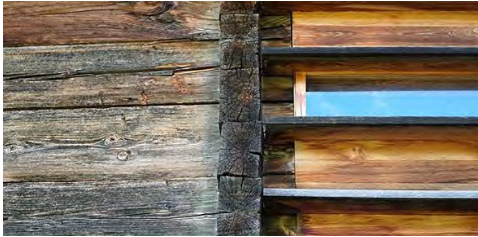
Facade detail, Gugulun House, Peter Zumthor
