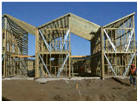
Villa Verde Housing, ELEMENTAL, under construction
