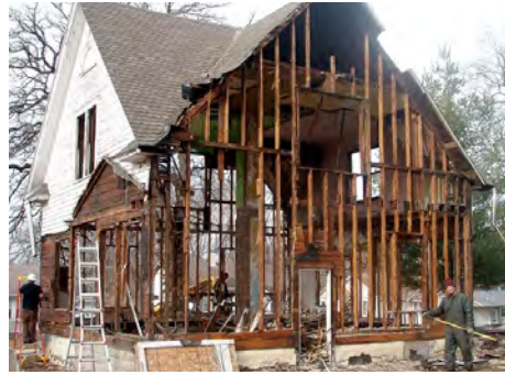
HUD deconstruction project, Detroit, MI
